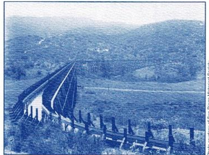
Los Coches Flume photo dated 1898
