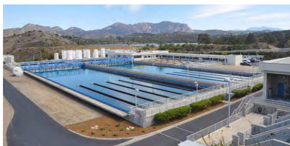
Figure 5.2 Helix Water District’s R.M. Levy Water Treatment Plant
