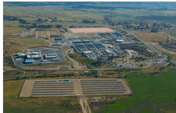
Figure 5.1 MWD’s Robert A. Skinner Water Treatment Plant
