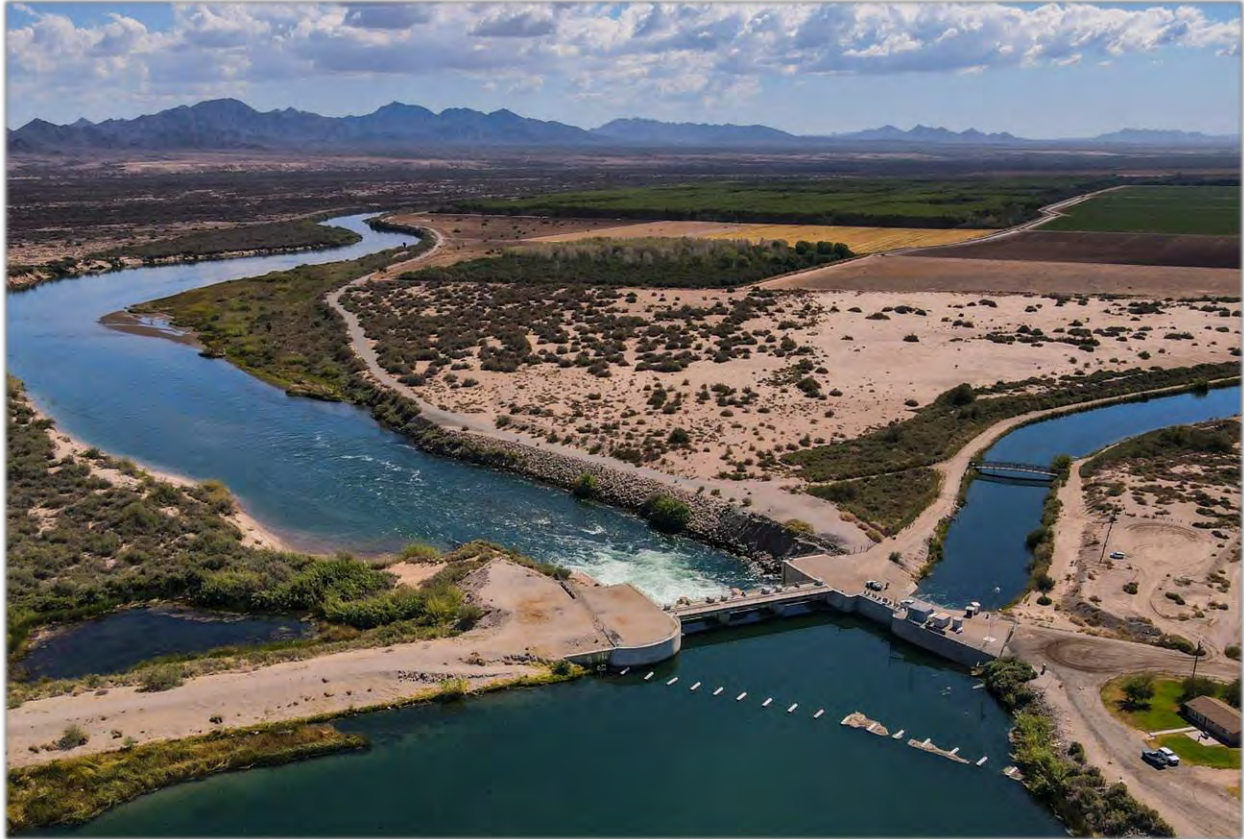
Figure 7.6 The Palo Verde Diversion Dam on the Colorado River
