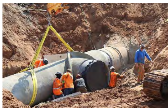
Figure 4.1 Installation of Large-Diameter Pipe for New Chet Harritt Pump Station
